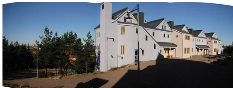
Fig. 2. The Rudolf Steiner School in Göteborg is an example of a three story building that employs this relatively simple ventilation system. Energy consumption for heating and electricity usually amounts to between 80-120 kWh/m 2 in buildings with the basic type of climate system.
