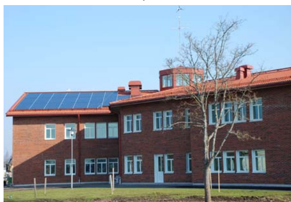
Fig. 10 Solar cell installation at Vargbro School.
